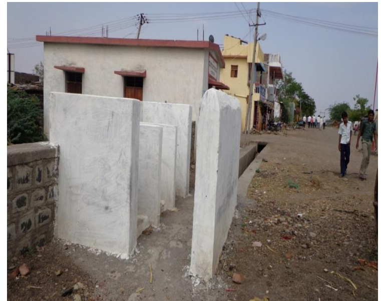
Public toilet constructed
