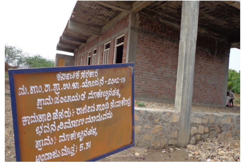
Rajiv Gandhi Seva Kendra under Construction
