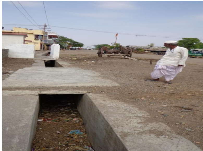
Drainage channel constructed
