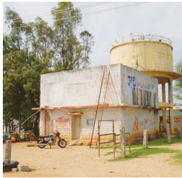
The village's source of potable water.
