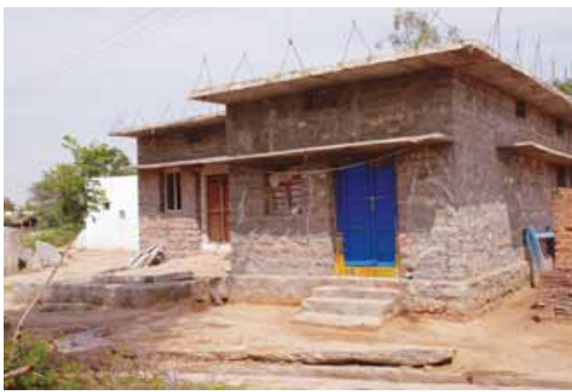
Subsidies are given for constructing houses.
